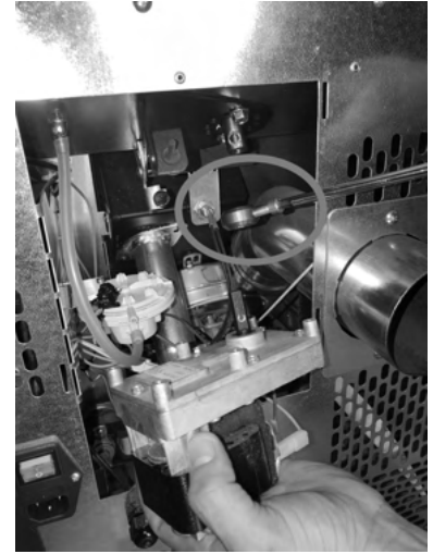
Fig. 80 - Gear motor removal
