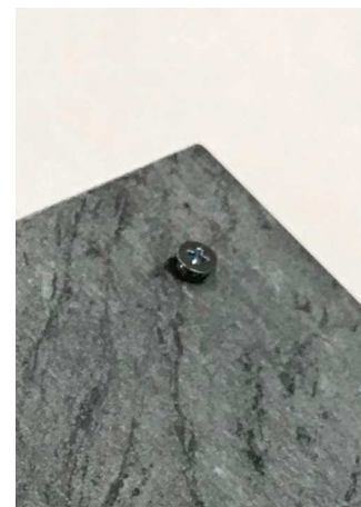
Fig. 37 - The screw must protrude
