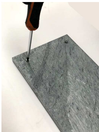
Fig. 36 - Tighten the screws
