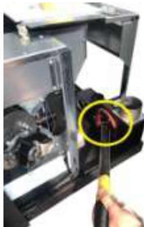
Fig. 115 - Smoke duct cleaning
