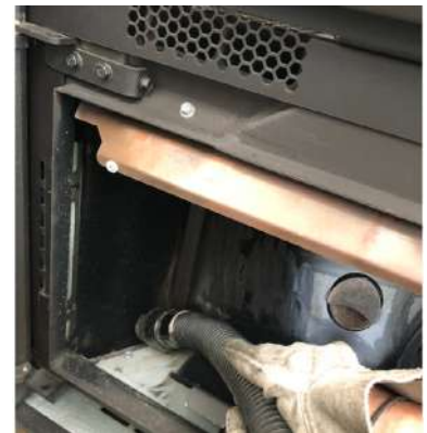
Fig. 108 - Vacuum out the ash
