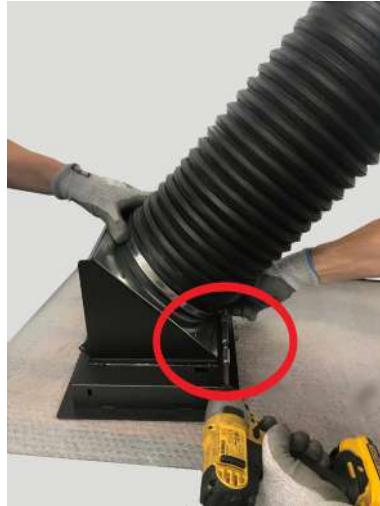
Fig. 65 - Tighten the clamp
