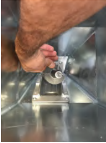
Fig. 94 - Spiral removal
