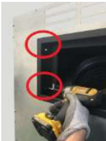
Fig. 70 - Trapdoor external fixing
