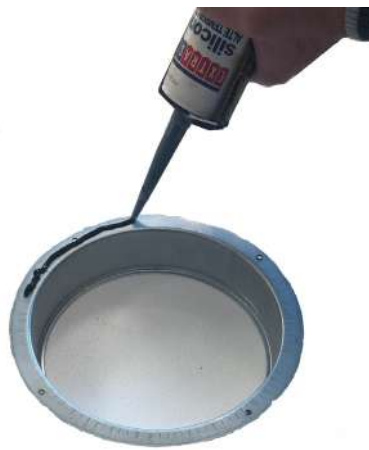
Fig. 68 - Silicone the flange
