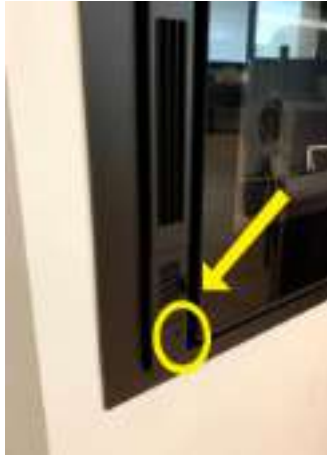
Fig. 29 - Thermostat probe
