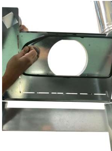
Fig. 54 - Gasket removal
