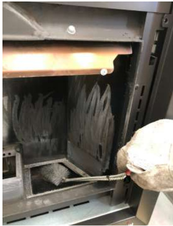
Fig. 104 - Clean with pipe cleaner
