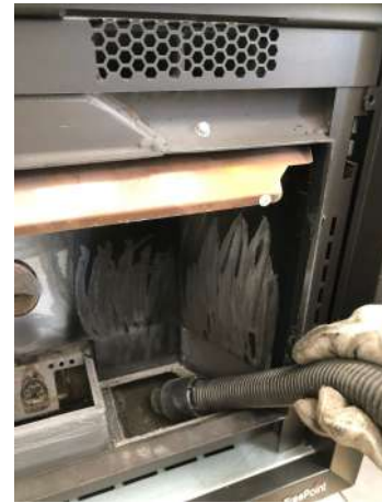
Fig. 105 - Vacuum out the ash
