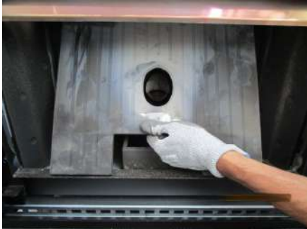
Fig. 112 - Central cast iron removal
