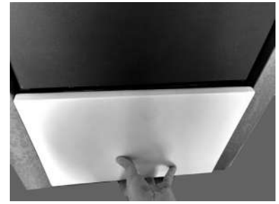
Fig. 25 - Hook the panel.
