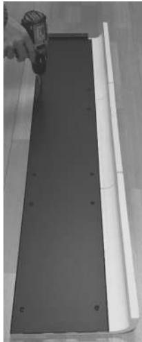
Fig. 26 - Fitting the maiolica panels
