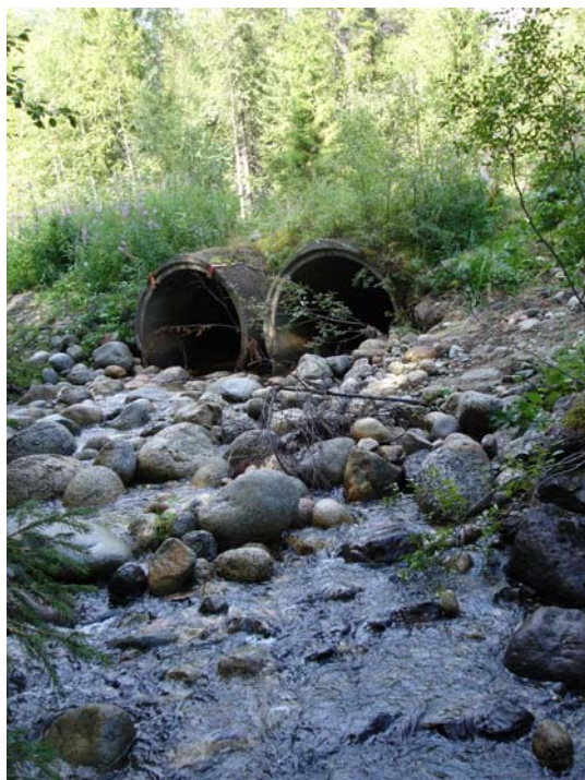
Figure 8. Improved road crossing in Tuggenbäcken by putting boulders downstream of the culverts.
