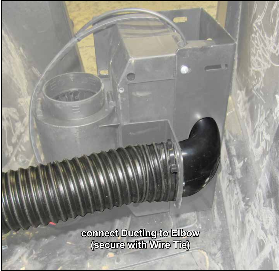
connect Tubing to Heater
