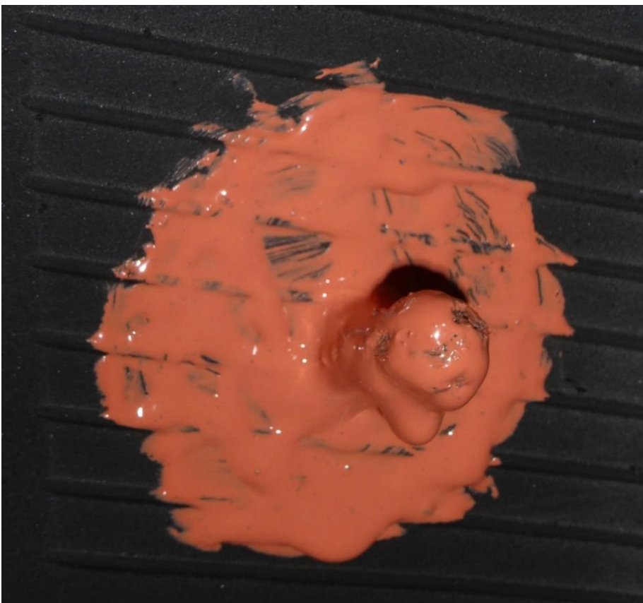
Liquid Patch was added and the repair area was sealed inside
