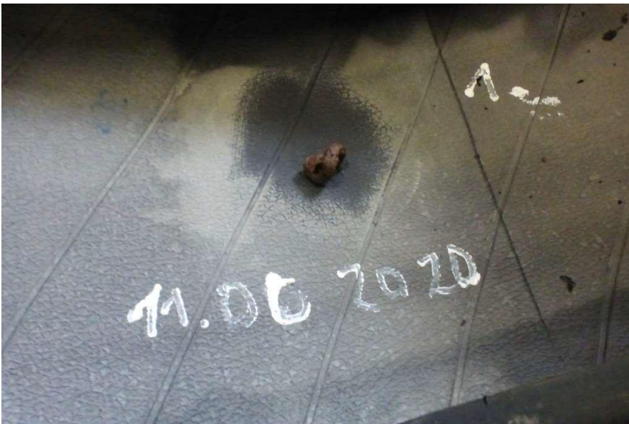
Cleaned repair site with inserted Safety Seal string. Date of manufacture 11.06.2020
