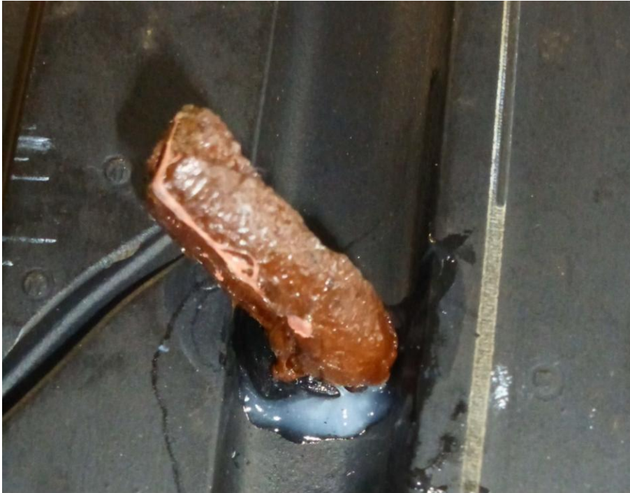
The hole channel has been closed with Material Safety Seal self Vulcanizing / String
